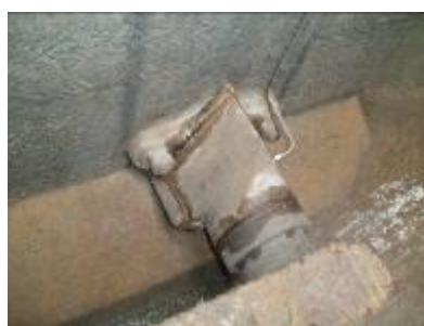
Peak cap bearing for Sedimentation Tank in Sewage treatment plant.
